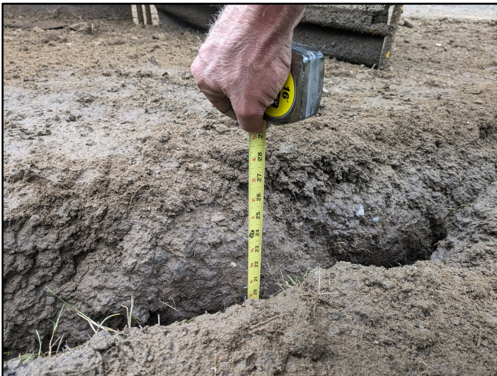
Photograph 3. Measuring trench depth.
