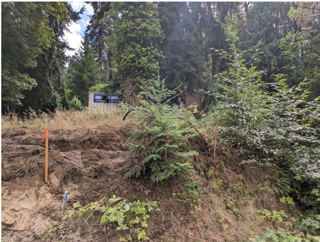
Photograph 5. The open trench north of tree 1005 above the existing slope. This slope is likely the result of a historic grade-cut.
